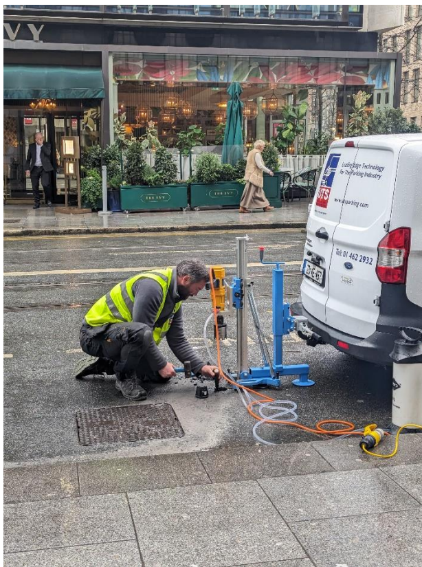
Figure 40: Sensor Installation on the loading bays
